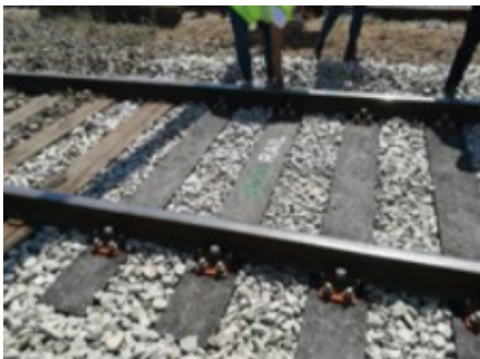
1st deployment completed in access line, at Entroncamento
