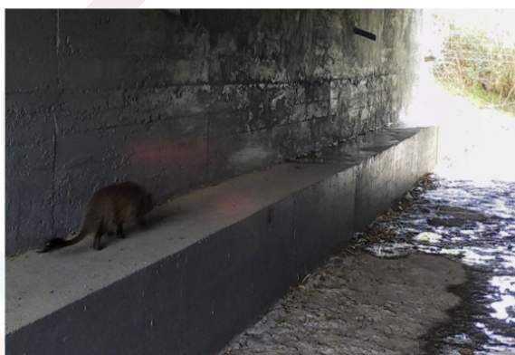
Wild carnivores fauna using causeways on Hydraulic Crossings and Engineering works (source: University of Évora)
