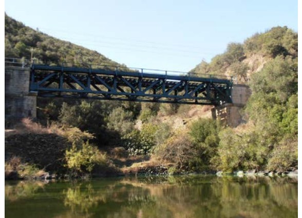
Metallic Structures on Beira Baixa Line
