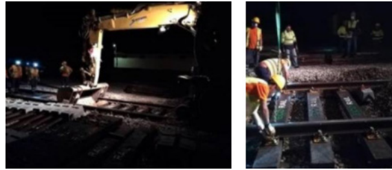
Replacement of wood sleepers by Eco Rail sleepers.
