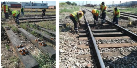
Deployment of the sleepers in access line, at Entroncamento
