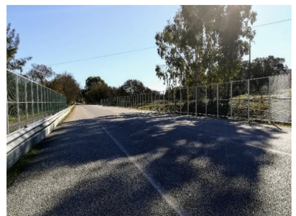
Installation of barriers to make night birds fly higher and thus prevent them from being run over
