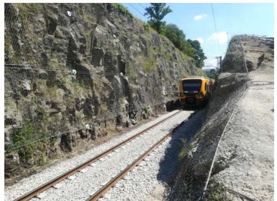
Douro Line Slopes
