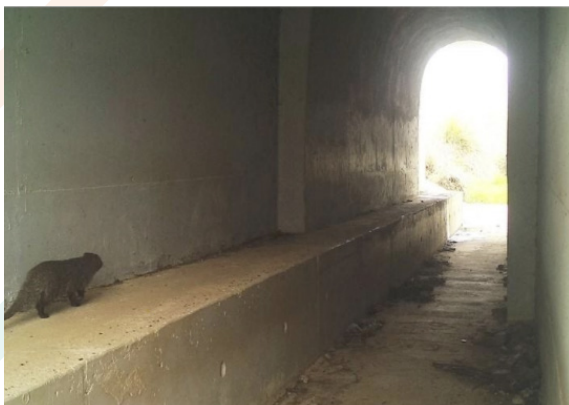
Wild carnivores fauna using causeways on Hydraulic Crossings and Engineering works (source: University of Évora)
