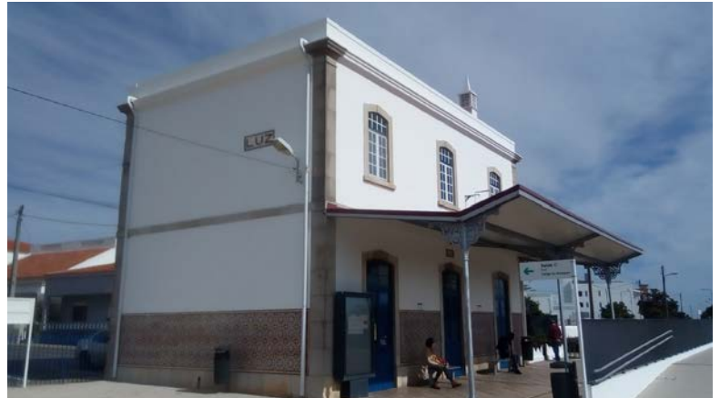
Renovation - Luz railway station
